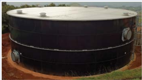
Trough Deck Roof
