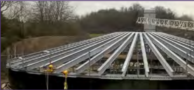
3: External Beam Roof – Anaerobic Digestion & Biogas
