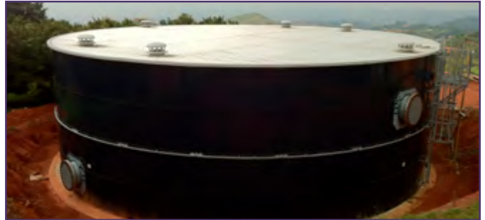
4: Trough Deck Roof – Drinking Water
